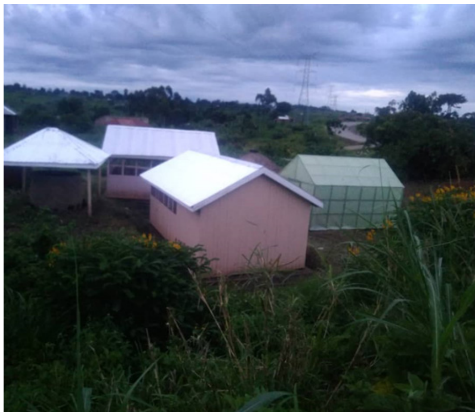
Constructed structures at Kyenjojo briquettes making and briquettes solar drier Project in Kyenjojo district
