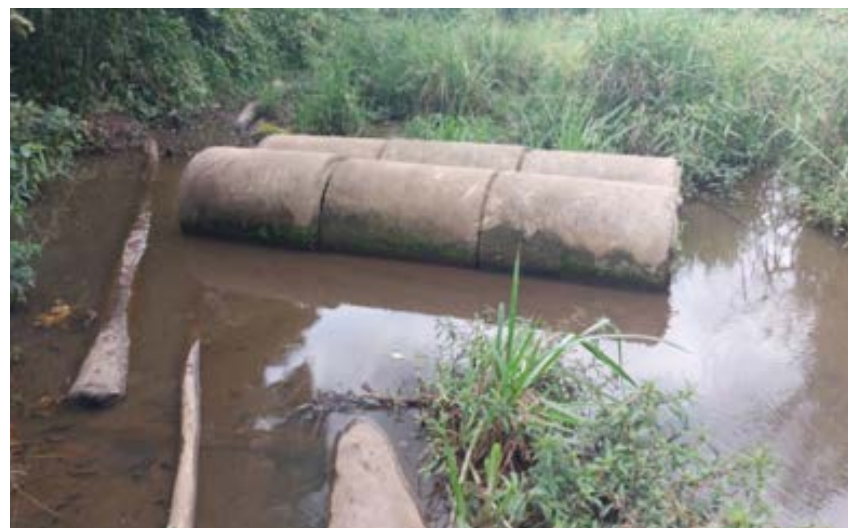
Figure 5: The culverts were donated by the political aspirant to garner support from the community
