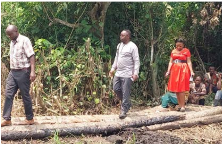
Figure 4: This is the only road the community relies on broken, unsafe, and long overdue for repair
