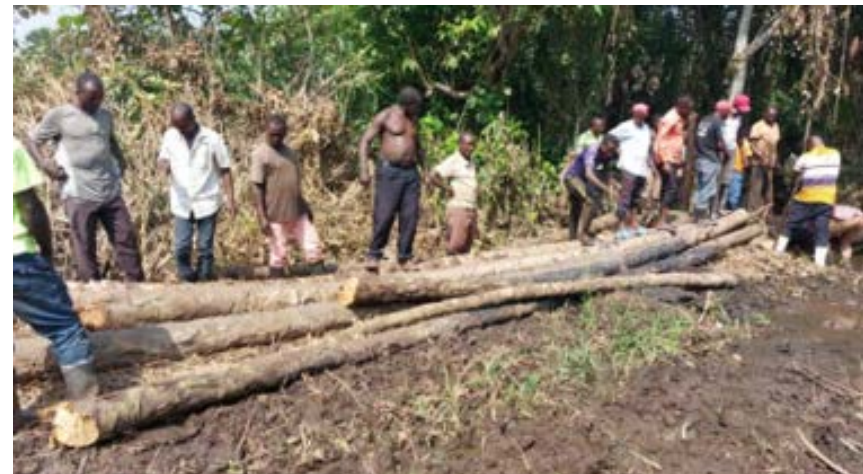
Figure 7: The community working together during the road construction
