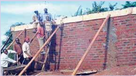
A store for Mahango Mambule Marketing Association at ring beam level and after roofing
