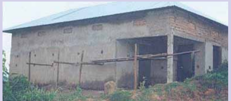
A store for Mahango Mambule Marketing Association at ring beam level and after roofing
